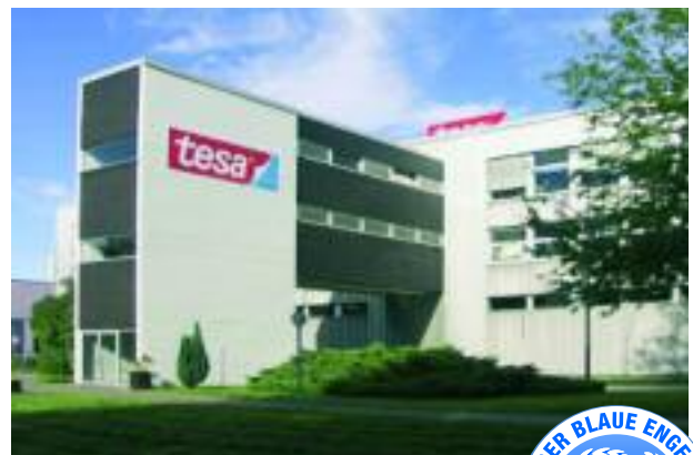
Certified tesa plant in Offenburg
